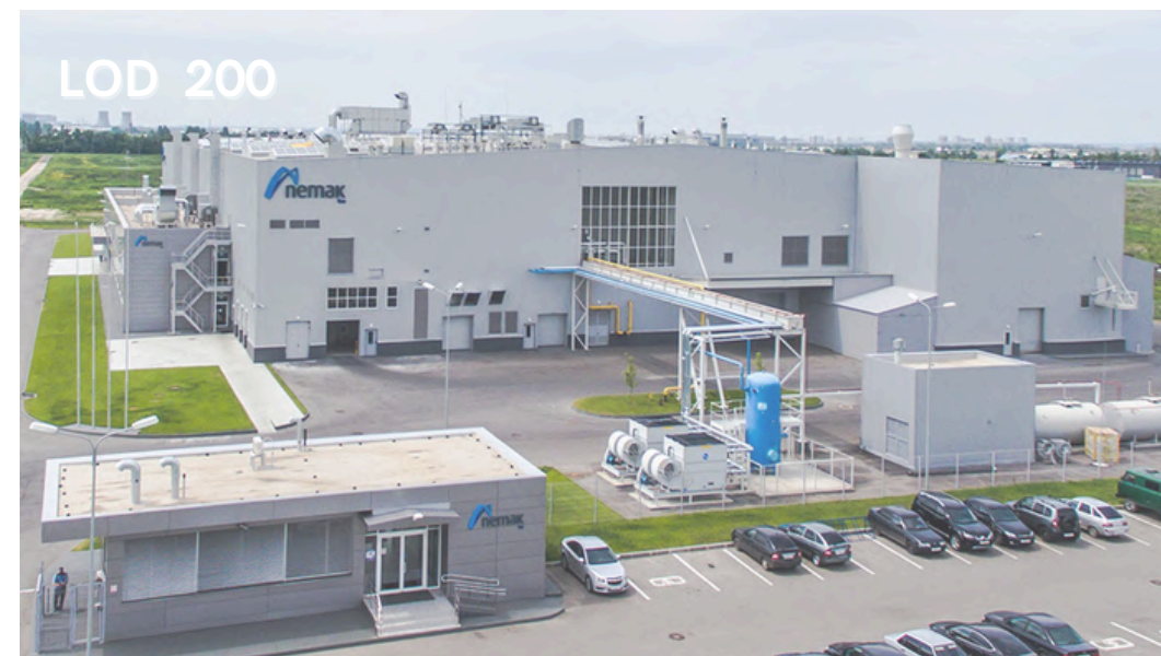
Nemak Factory Building, Ulyanovsk, Russia 12.000 m 2 , Architectural and Structural Projects
